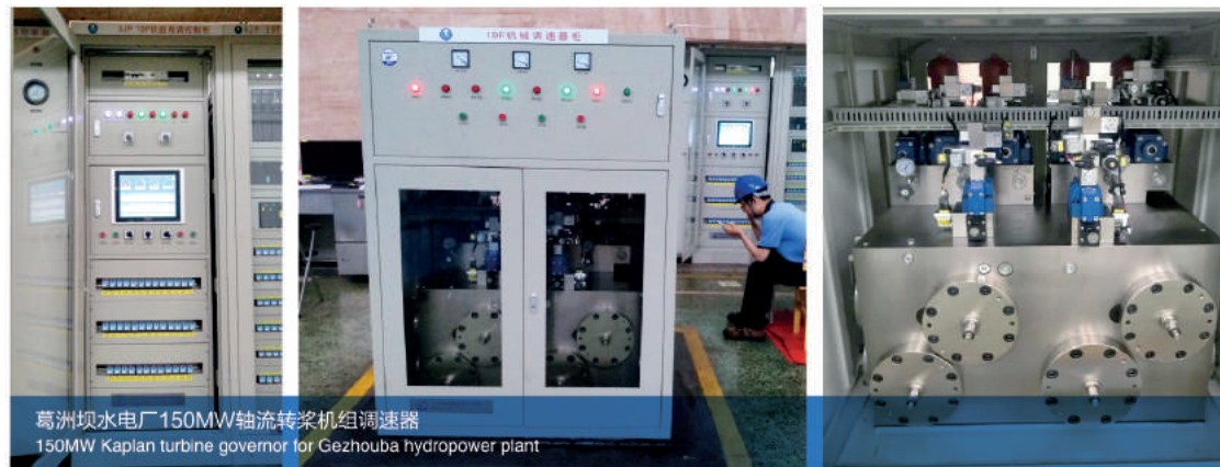
公伯峡水电站300MW混流机组调速器 300MW Francis turbine governor for Gongboxia hydropower plant
